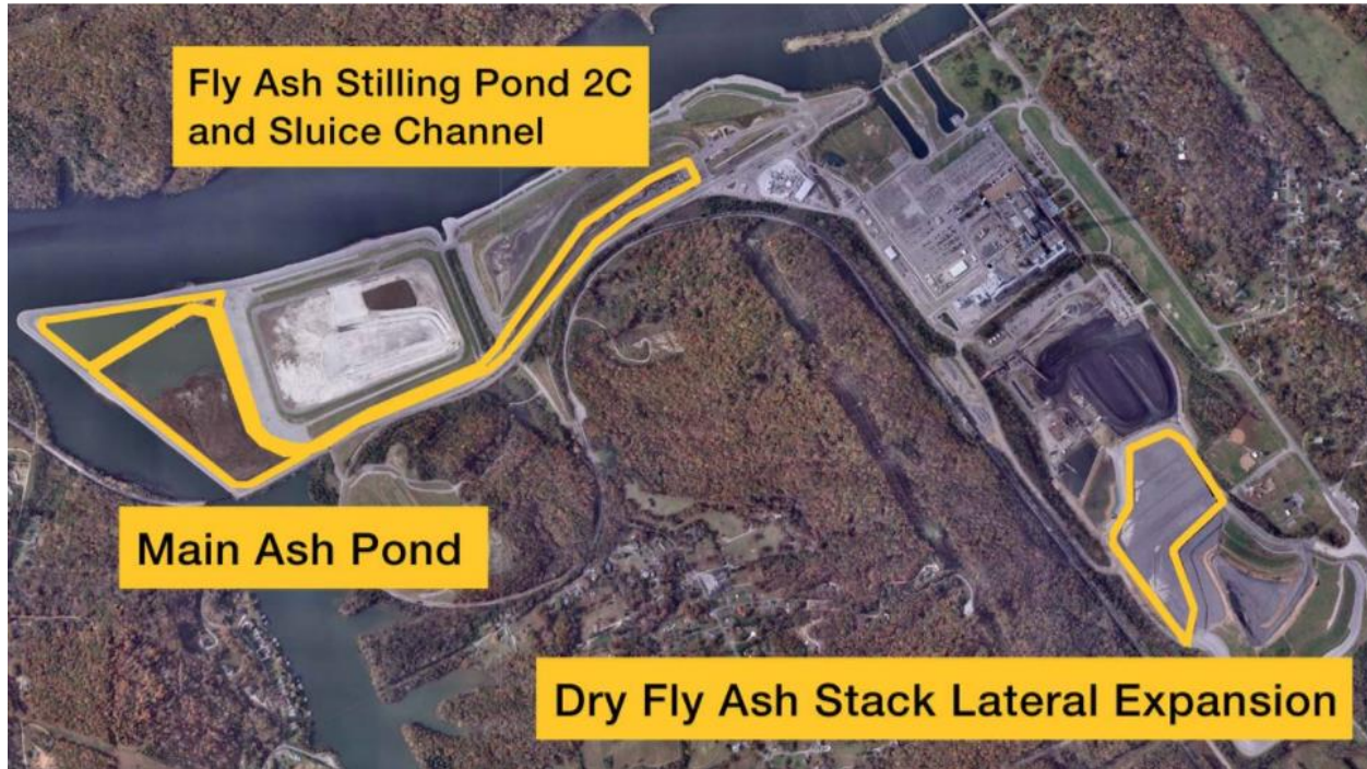
Figure 1: Aerial View of Ash Pond Complex
