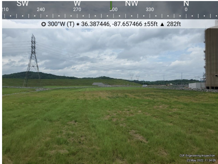
Photo C-1 View of the Bottom Ash Pond. General conditions, no deficiencies observed.
