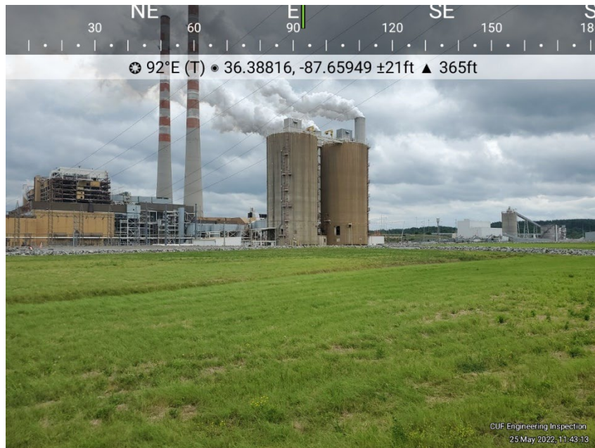
Photo C-2 View of the Bottom Ash Pond. General conditions, no deficiencies observed.
