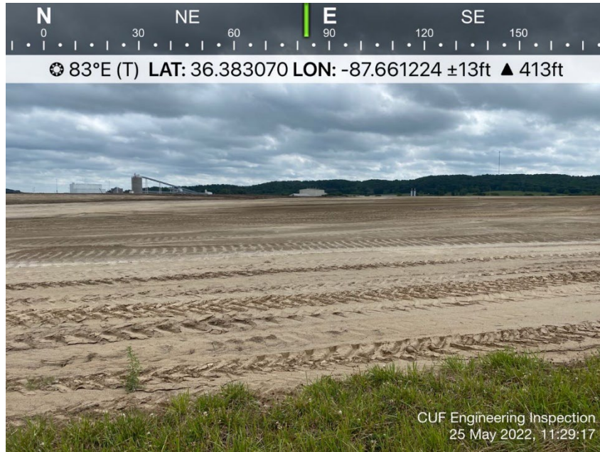
Photo D-1 View of top interior of the Gypsum Storage Area. General conditions, no deficiencies observed.
