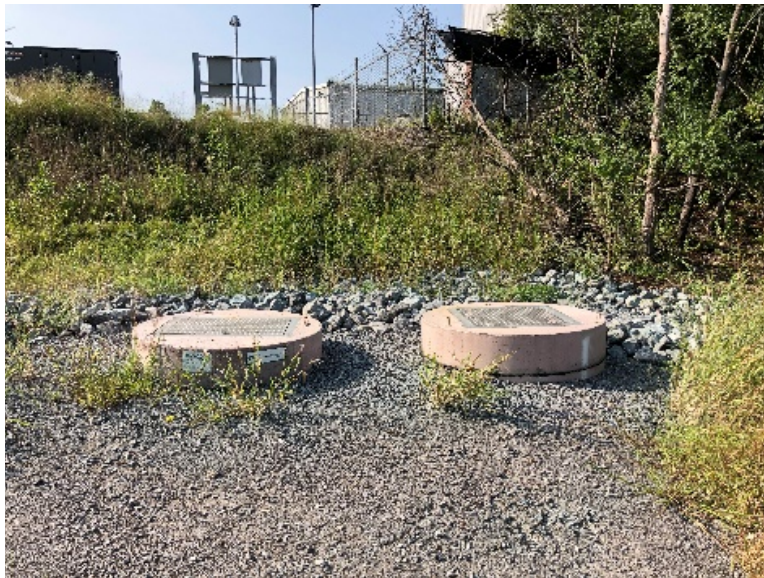
Photo 2 Collection system at Seep 13 at Ash Pond E. No deficiency pictured.
