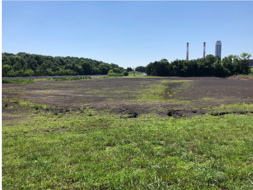
Photo 5 General view of Bottom Ash Pond looking south. No deficiency pictured.
