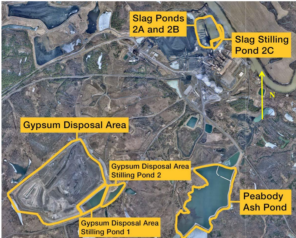
Figure 1: Aerial View of the Gypsum Disposal Area
