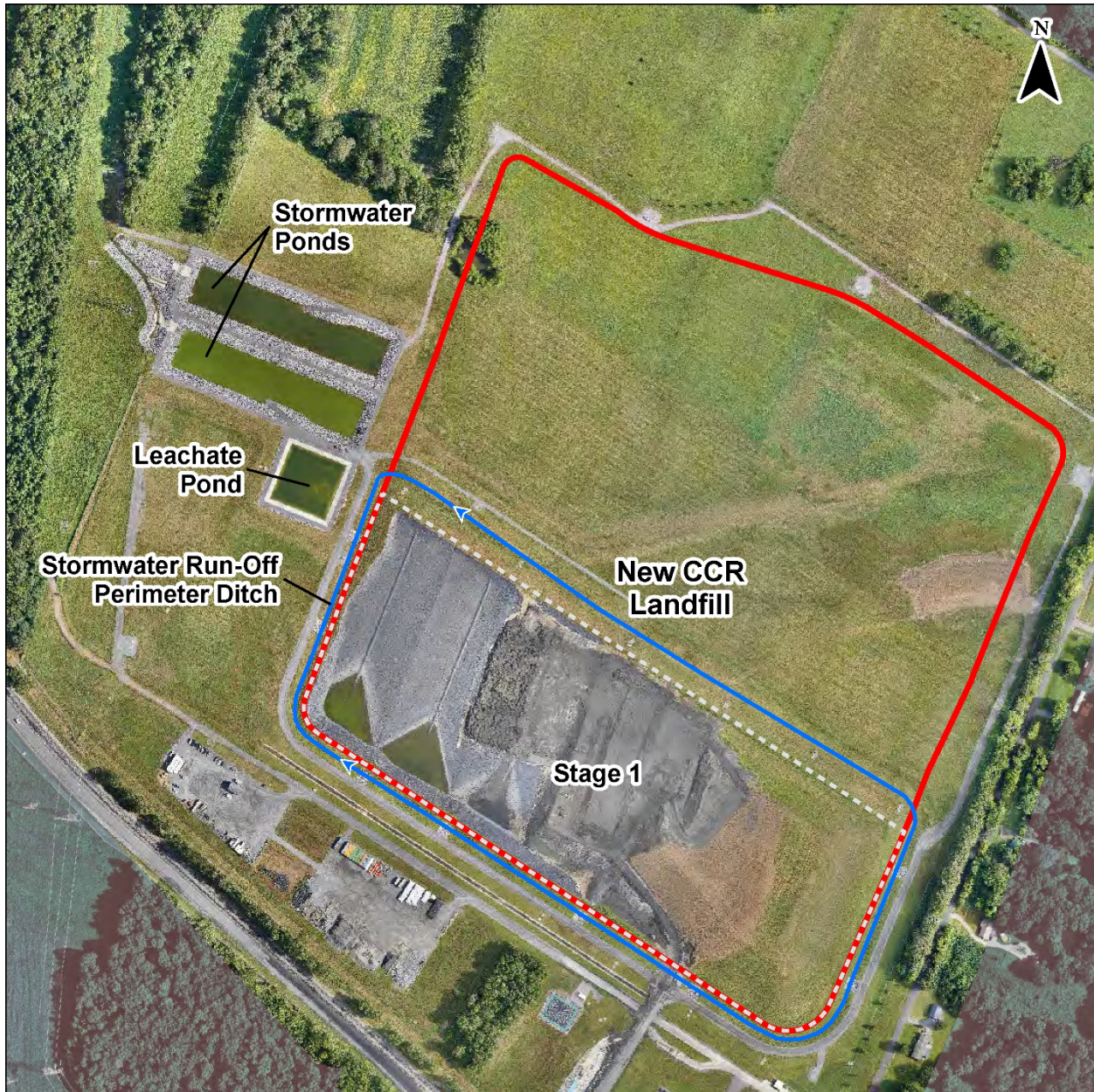
Figure 1. SHF New CCR Landfill – Current Conditions
